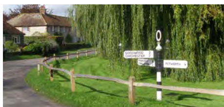
New single post and rail fencing around East Dean Pond and Green
